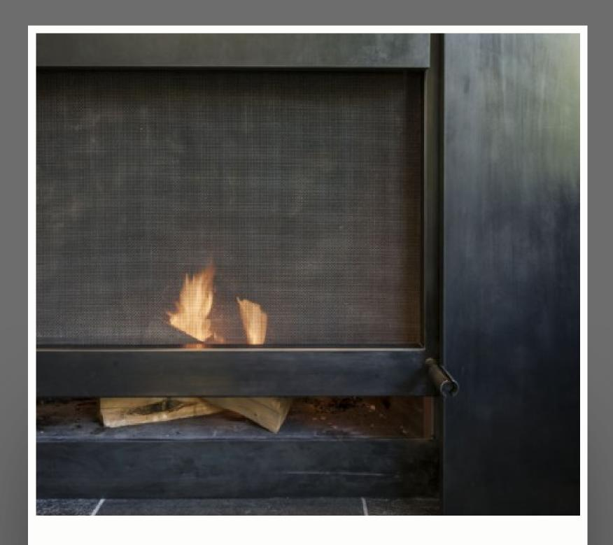
The Indian Springs Guillotine Fireplace and blackened steel surround is a perfect example of a contemporary use of patina'd steel. The steel panels are hand patina'd and hung on a steel frame with Z-clips so that there is a very concise tight joint. The fireplace door is a guillotine style screen that recesses up into the steel above. Clean lines and custom engineering.
